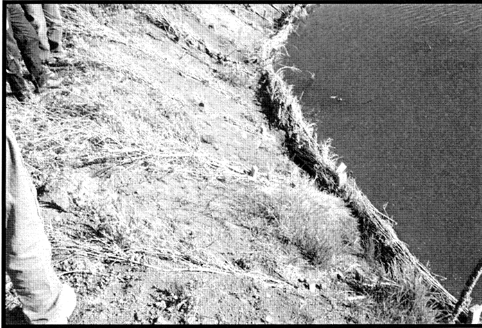
Figure 23. The Little Colorado River Enhancement Demonstration Project is using bio-engineering channel design approaches to restore a segment of the Little Colorado River. 99-092WPF
