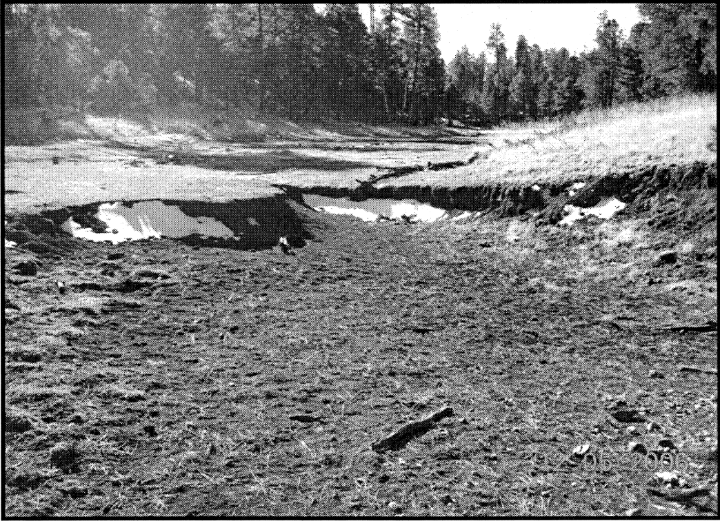
Figure 32. A degraded section of Fairchild Draw prior to restoration activities. 07-150WPF
