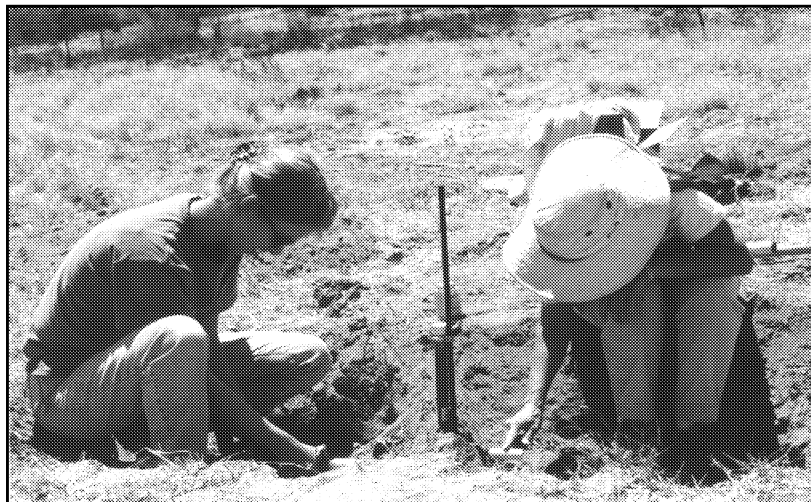
Figure 18. Rincon Institute Staff installing irrigation control valves at the Llewellyn revegetation site. 98-062WPF
