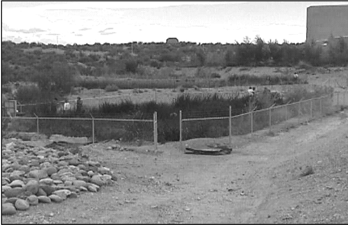
Figure 22. Portion of the wetland facility at Wickenburg High School. 99-088WPF
