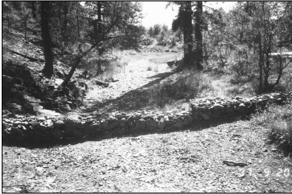
Figure 8. Erosion Control Structure at Mingus Springs Camp. 96-0007WPF
