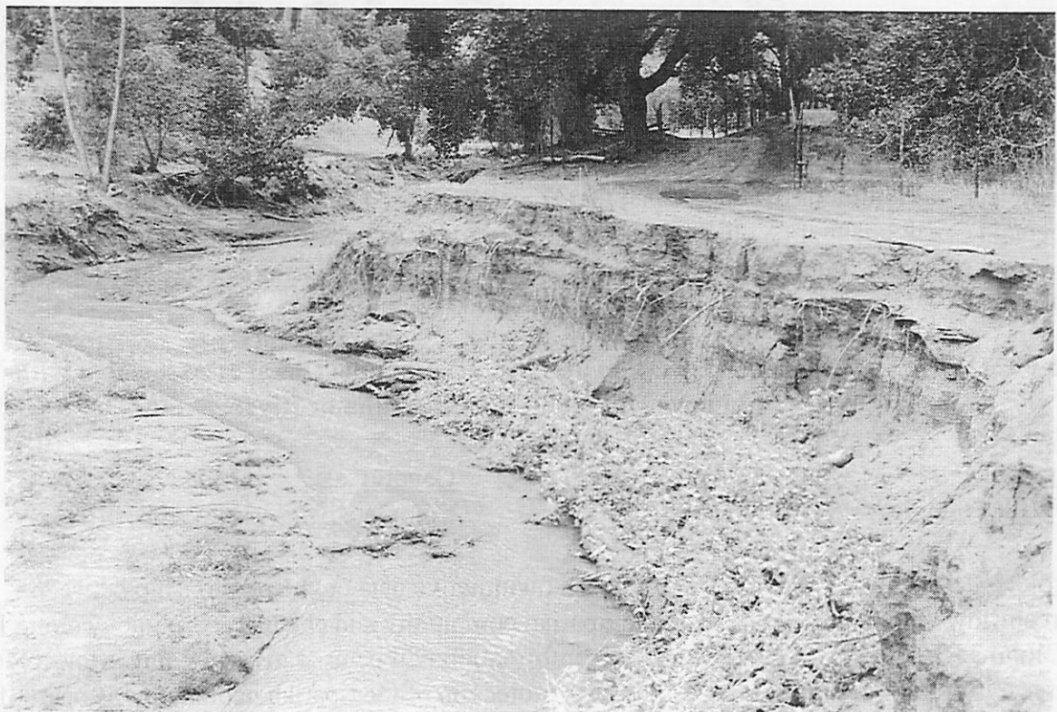
Figure 11. Site of potential road failure due to bank erosion, Canyon del Muerto. 96-0025WPF.
